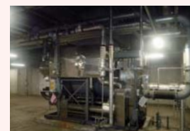
Steam-driven absorption refrigerating machine (1,050 kW)
