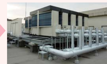
High-efficiency air-cooled heat pump module chiller (150 kW x 7 units, made by Daikin)
